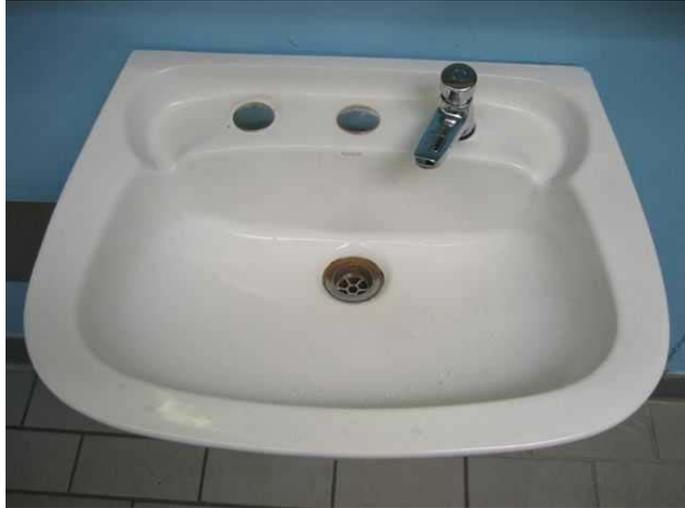
Figure 2: Photo of Enware timer push-button taps on hand wash basins in female change rooms.
