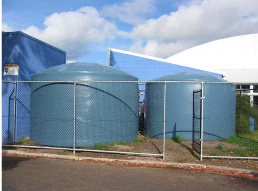
Figure 1: Photo of rainwater tanks (2 x 31,500 litres) providing potable water to the Jubilee Park Aquatic Centre for drinking and hygiene purposes.
